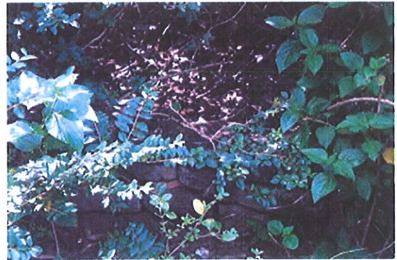
22. Dry-stone wall to adjacent tank/ boundary.
