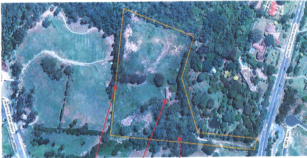
5. Recent aerial -detail. Trees to boundary, cottage, remnant vegetation (Source: www.imagery.maps.nsw.gov.au )
