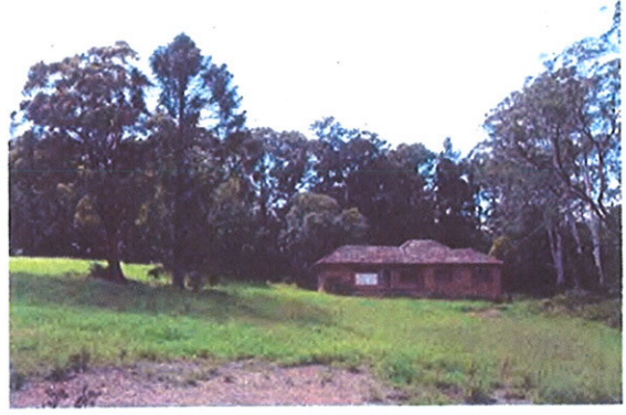
14. Cottage and Bunya from the west.
